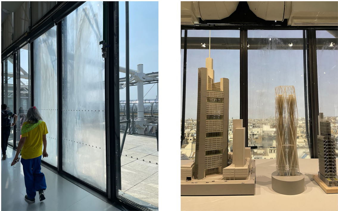
Fig. 1 Effect of condensation in the IGU cavity on the transparency of the glazing; Centre Pompidou, Paris
