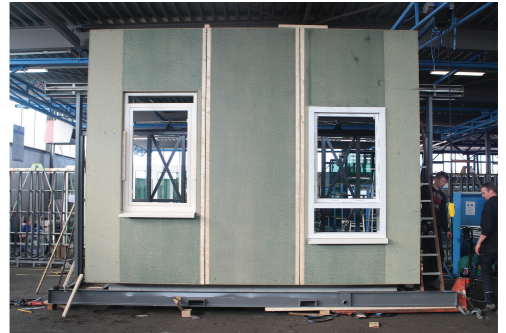
Mock-Up: Prefabricated facade elements
