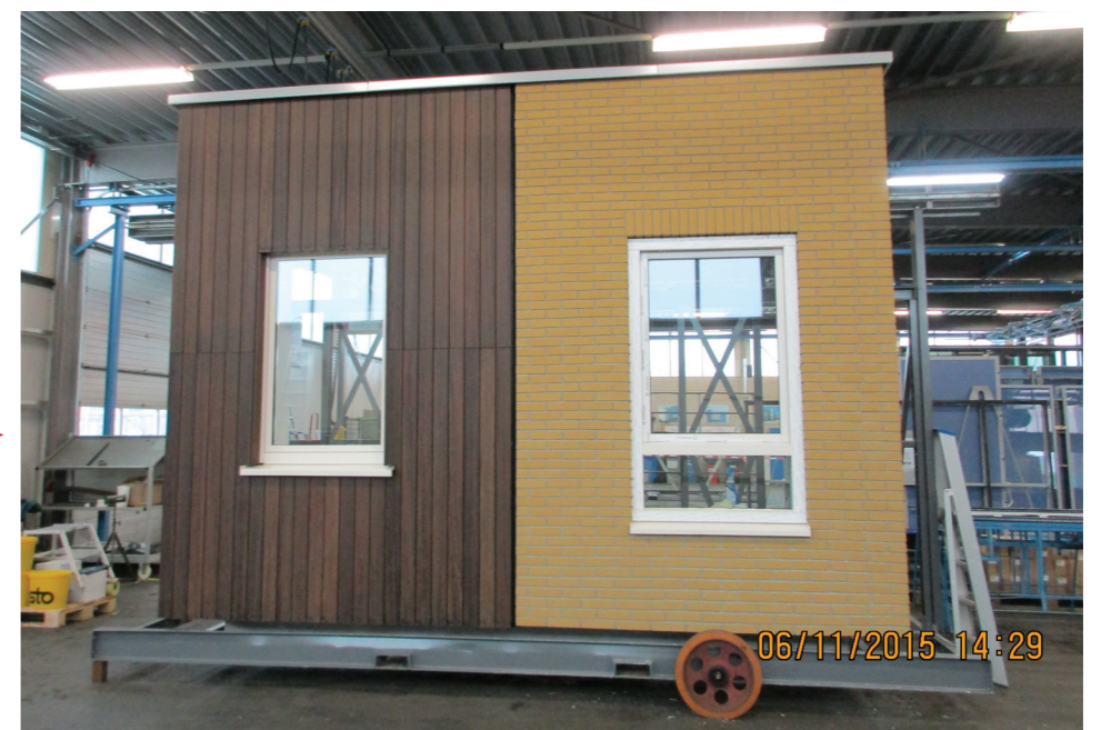
Mock-Up: Bamboo cladding (left); brick cladding (right)
