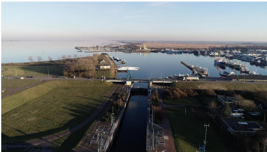
Figure 14: View of the Goereese Sluis and the waiting port
