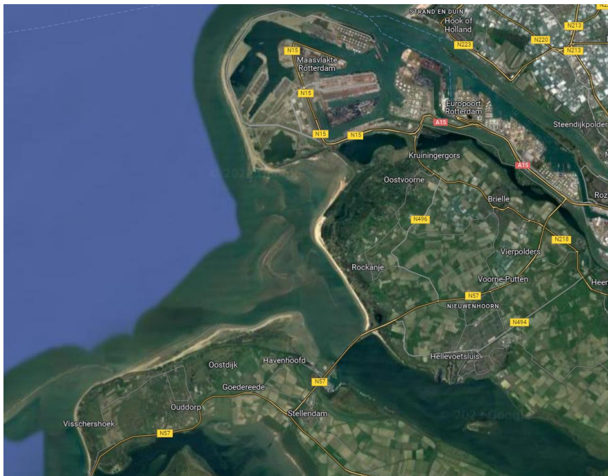
Figure 6: Current View of Haringvliet estuary (Google, 2022)
