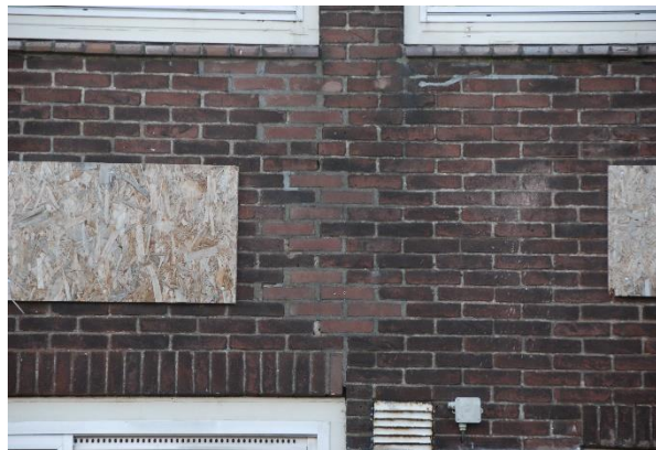
Figure 111: Previous Test Location Detail 1
