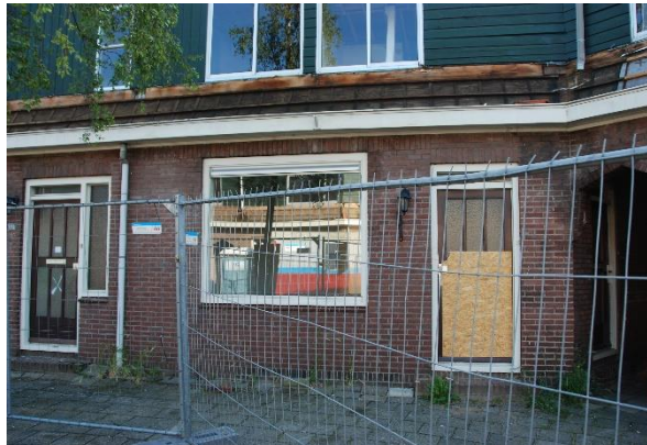
Figure 97: Location 1: Front View
