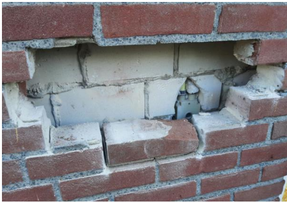
Figure 118: Location 1 Brick 3 overview
