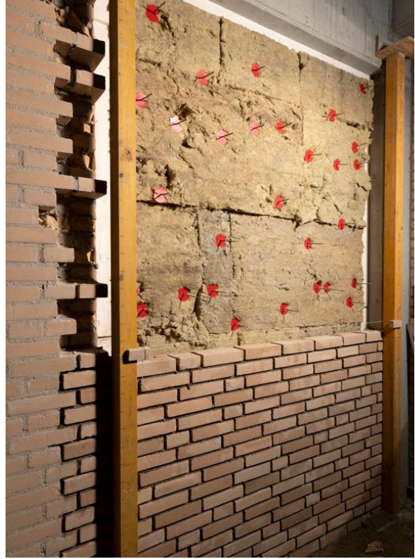
Figure 42: Bricklaying the Inner Wall
