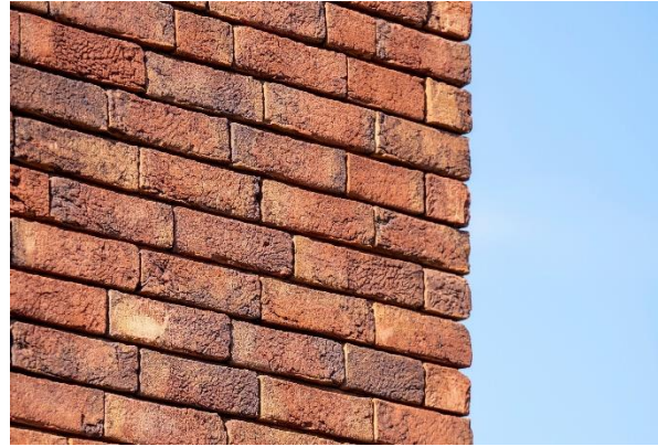
Figure 2: Final Look Drystacking (Wienerberger, 2024)
