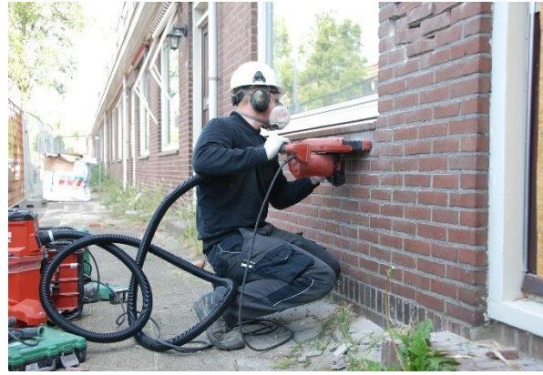
Figure 128: Location 1, upper saw cut
