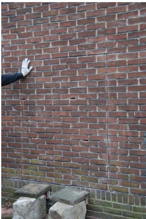
Figure 144: The cut element still in the wall
