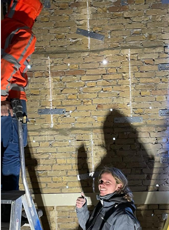
Figure 41: Results of added Mortar (horizontal) and Joint Sealer (vertical).
