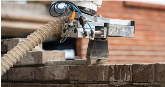
Figure 3: Robot Applying Mortar (Ballast Nedam, 2022)
