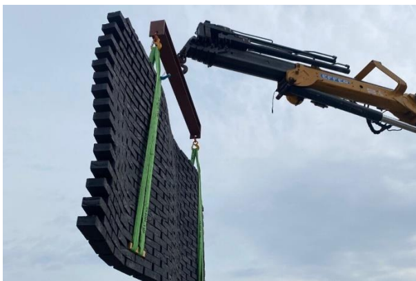
Figure 5: Prefab Masonry Lifted (Vekemans, 2023)
