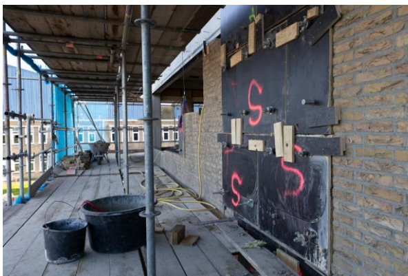
Figure 39: Masonry Elements are put in Place
