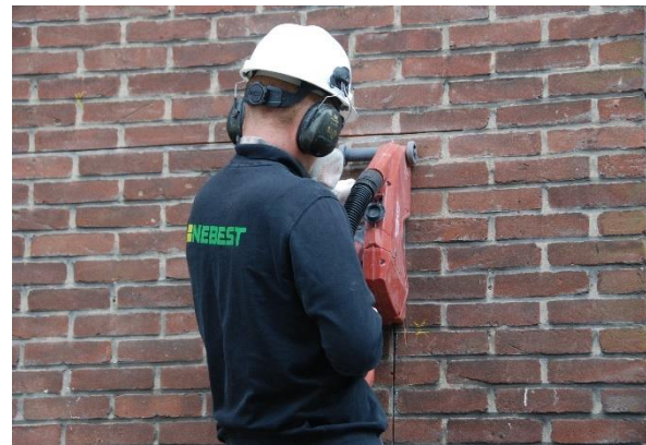
Figure 141: Vertical cut standing position
