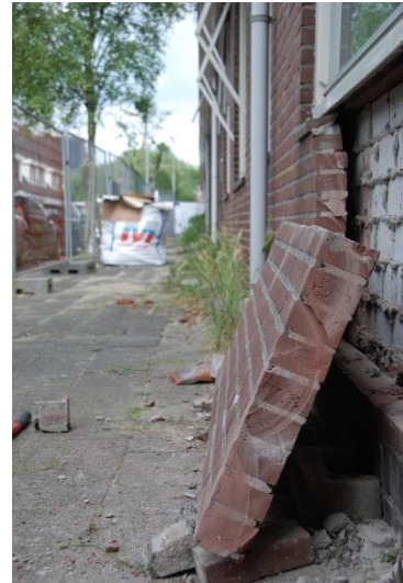
Figure 143: Side view of masonry element
