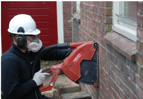
Figure 140: Vertical cut low position
