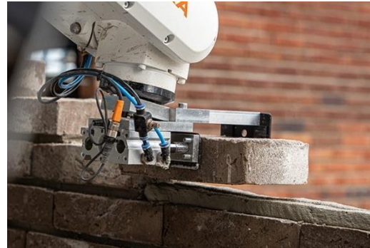
Figure 4: Robot Applying Brick (Ballast Nedam, 2022)
