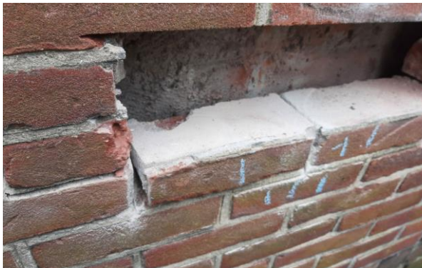
Figure 121: Location 2 Brick 1 Overview
