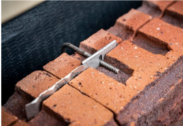
Figure 1: Drystacking Principle (Wienerberger, 2024)
