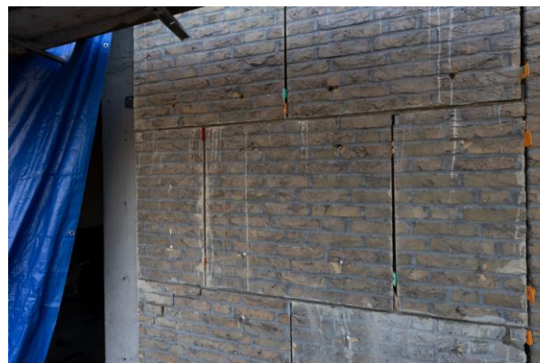
Figure 40: Preparations before adding Mortar
