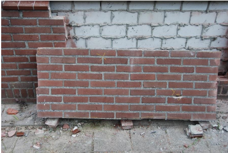
Figure 142: Element resting on 3 bricks
