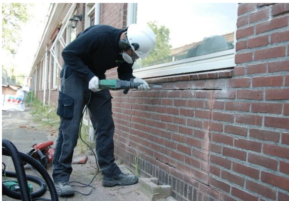
Figure 129: Removal row above element
