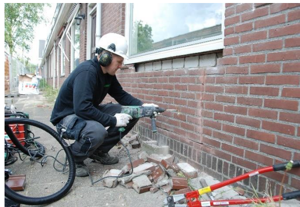
Figure 130: Removal row above finished
