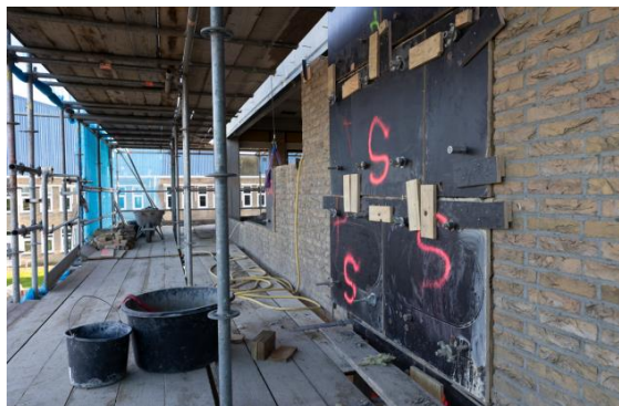
Figure A 9: Masonry elements in wall @VINK Bouw
