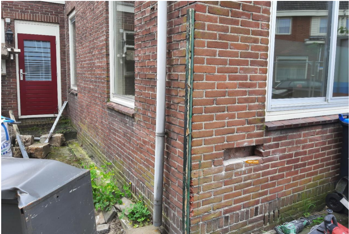
Figure 120: Location 2 Destructive Test Location
