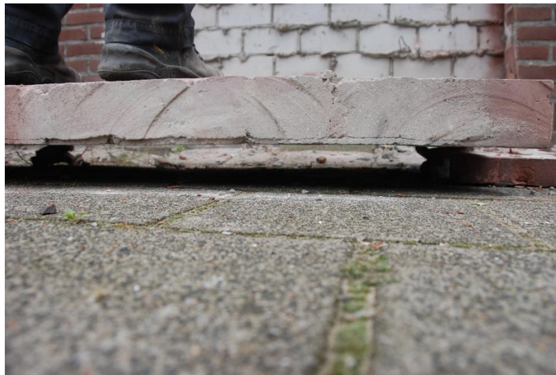
Figure 151: View under the masonry element of location 1
