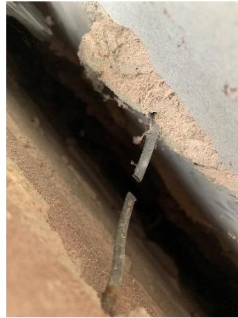
Figure 135: Wall tie cut
