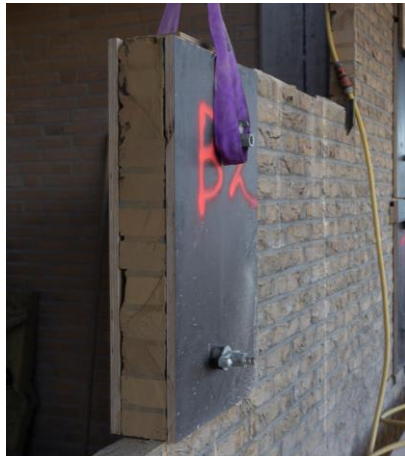
Figure A 4: Hoisting by lifting straps @VINK bouw
