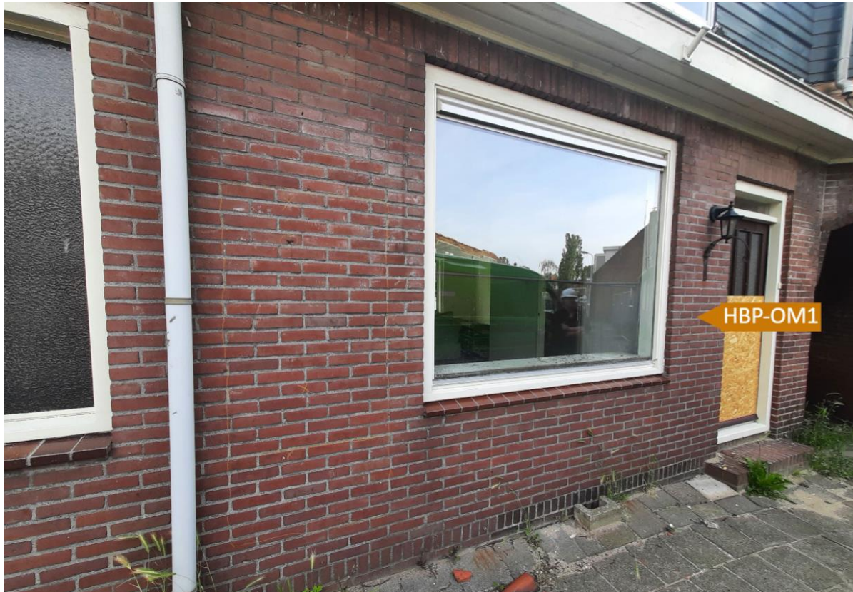
Figure 113: Location 1 Destructive Test Location
