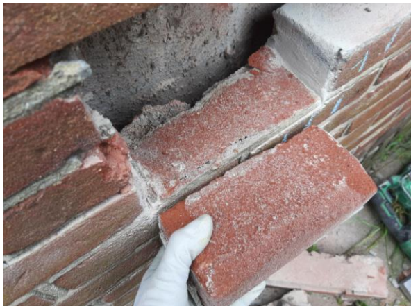
Figure 123: Location 2 Brick 2 Overview
