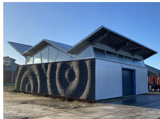
Figure 6: Prefab Masonry on Location (Vekemans, 2023)
