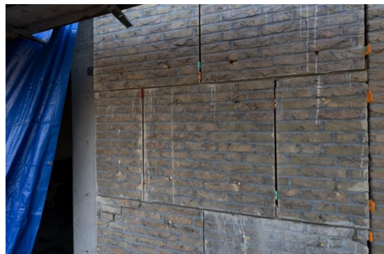
Figure A 10: Masonry element in wall @VINK bouw
