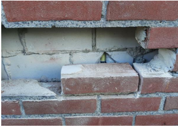
Figure 116: Location 1 Brick 2 Overview
