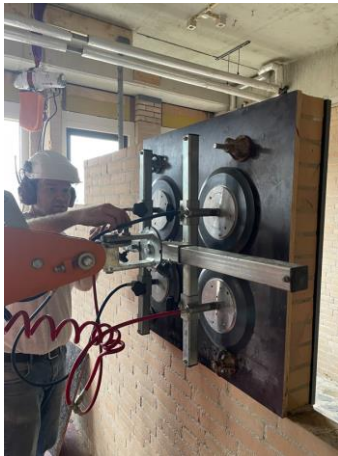
Figure A 3: Hoisting by glass lifter @VINK bouw
