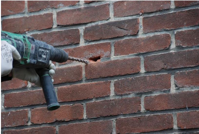
Figure 138: Drilling to remove wall ties
