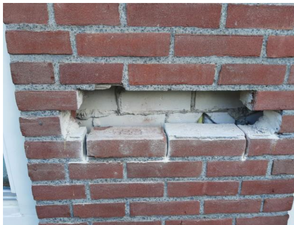
Figure 114: Location 1 Brick 1 Overview
