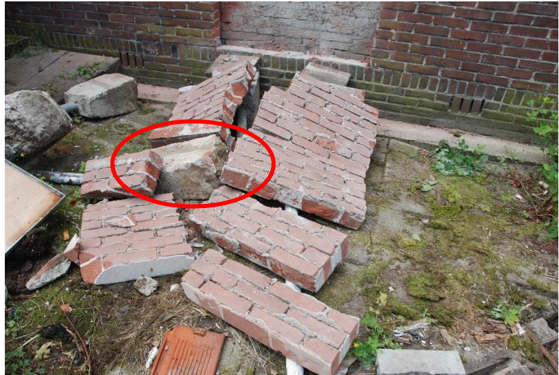
Figure 153: The reason element 2 brock apart
