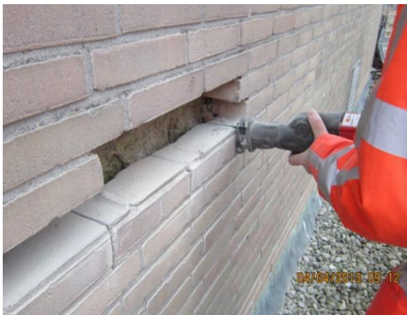
Figure 22: Removing Masonry Joints @nebest
