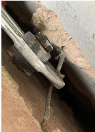
Figure 134: Small bolt cutter around wall tie
