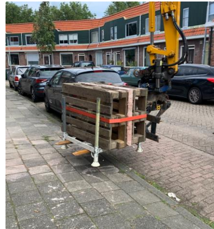
Figure A 5: Hoisting by forklift
