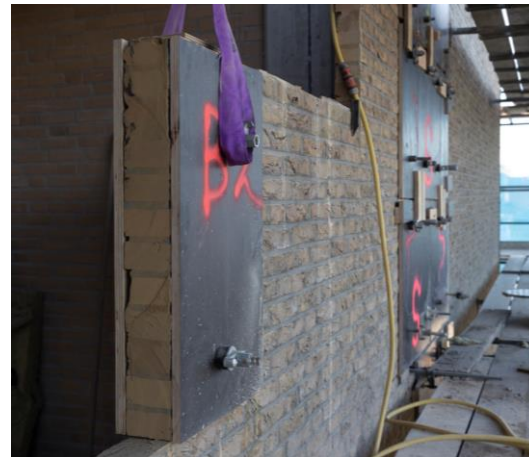
Figure 32: Hoisting by Lifting Straps by Vink B.V.
