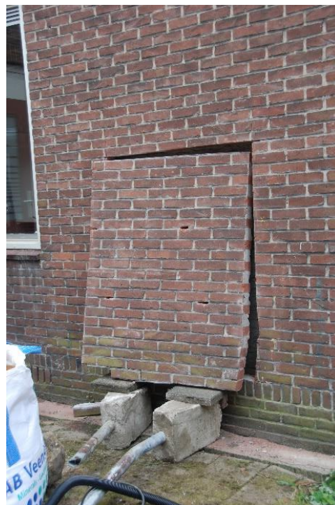
Figure 145: Element removed from the wall
