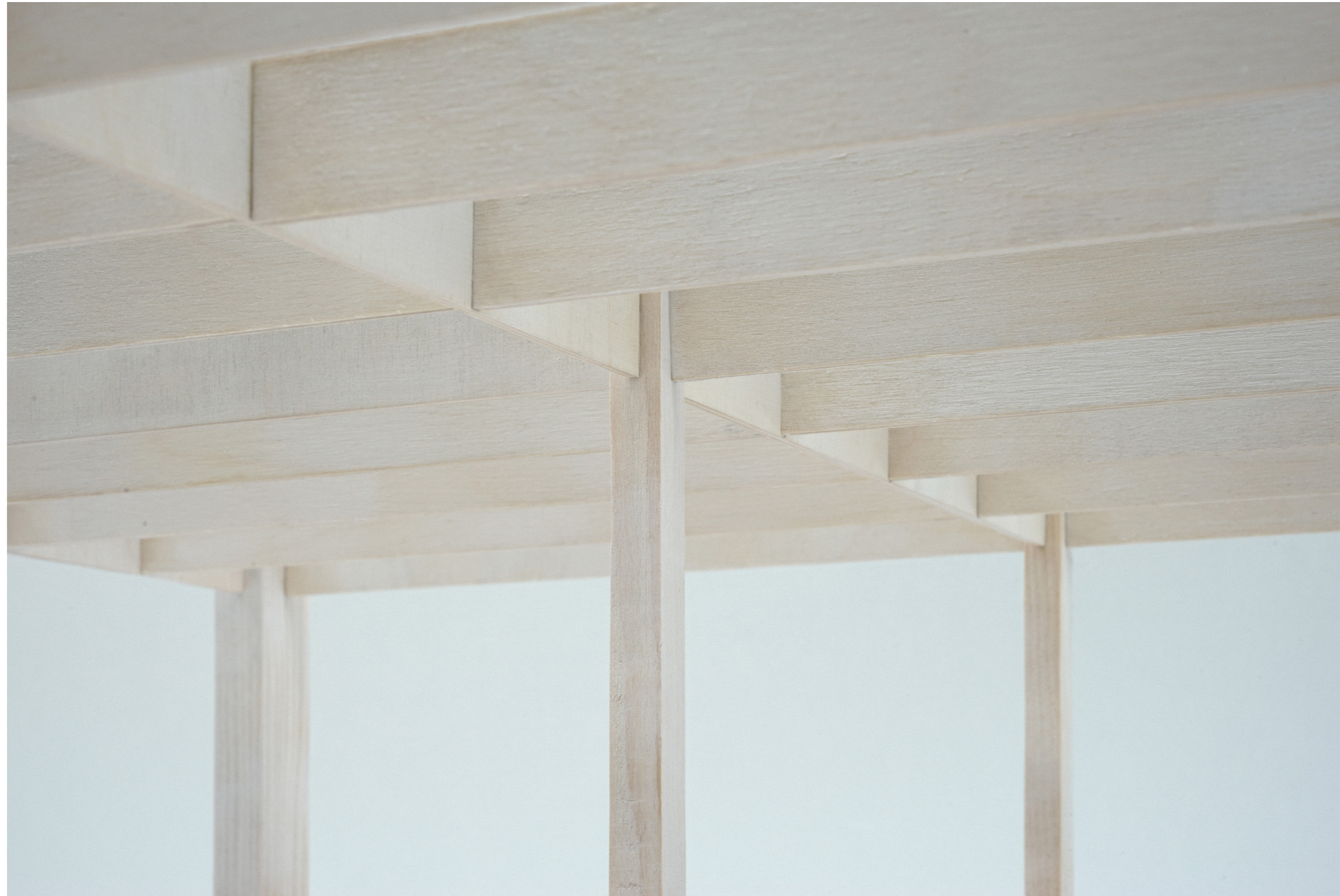
Primary Timber Structure – Glue-Laminated Columns and Beams
