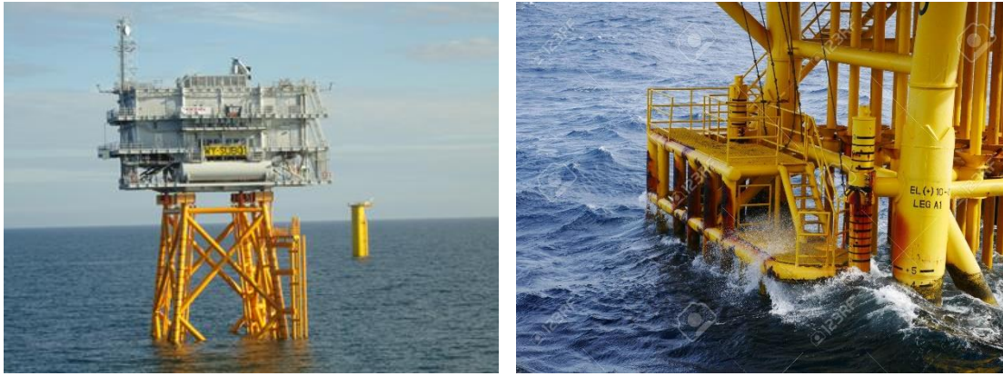
Figure 5.6 – Jacket with boat landing [36][37]
