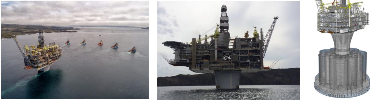
Figure 5.8 – Images of GBS (Exxon Mobil's Hebron) being towed and in- place [40]
