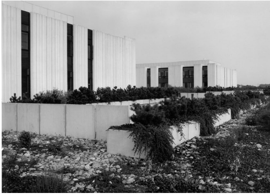
Hvidovre Hospital, Facade on the roof terrace, 1978 Source: Hvidovre Hospital Archive
