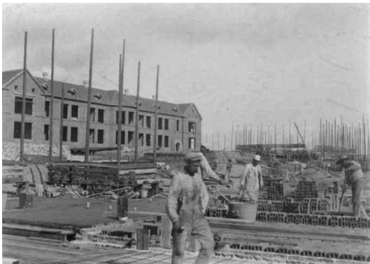
Bispebjerg Hospital, Construction Site, 1910s Source: Det Kongelige Bibliotek
