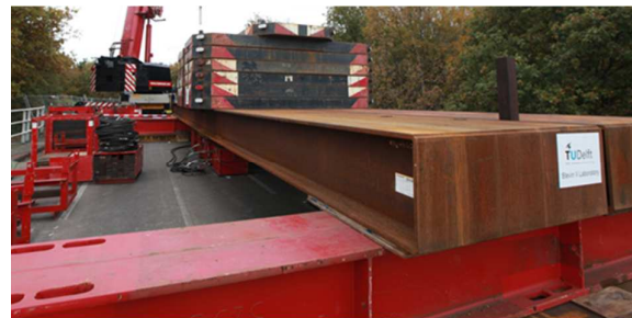
Figure 5. Loading system, showing load spreader beam, counterweights, and hydraulic jacks.
