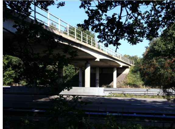
Figure 1. Viaduct de Beek
