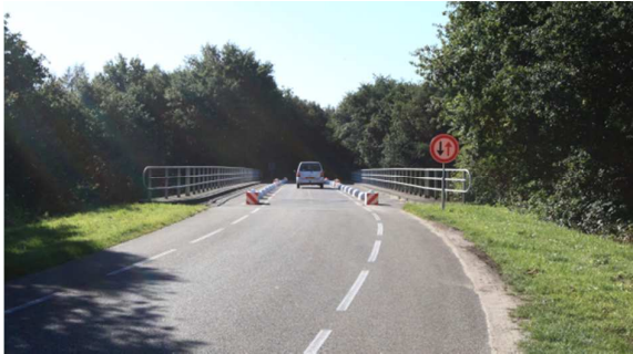
Figure 3. Traffic restriction on viaduct de Beek
