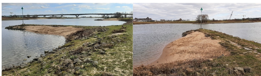
Figure 12. Natural streamlining of groynes along the Nederrijn River at Arnhem (km 880.4) by lee-side deposition of sand during floods. Photographs taken on 6 March 2021 after flood with 7,395 \text{ m}^3 \text{ s}^{-1} peak discharge at Lobith gauge station (approximate return period: 5 years) on 8 February 2021 (courtesy Tom Buijse).
