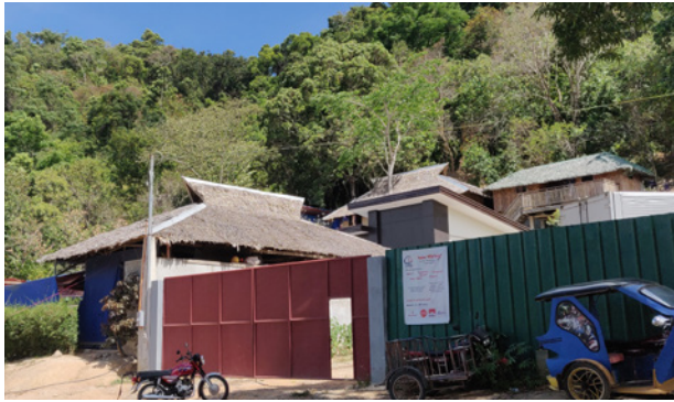
Figure 15: Roof made of reed with opening for stack effect, Palawan
