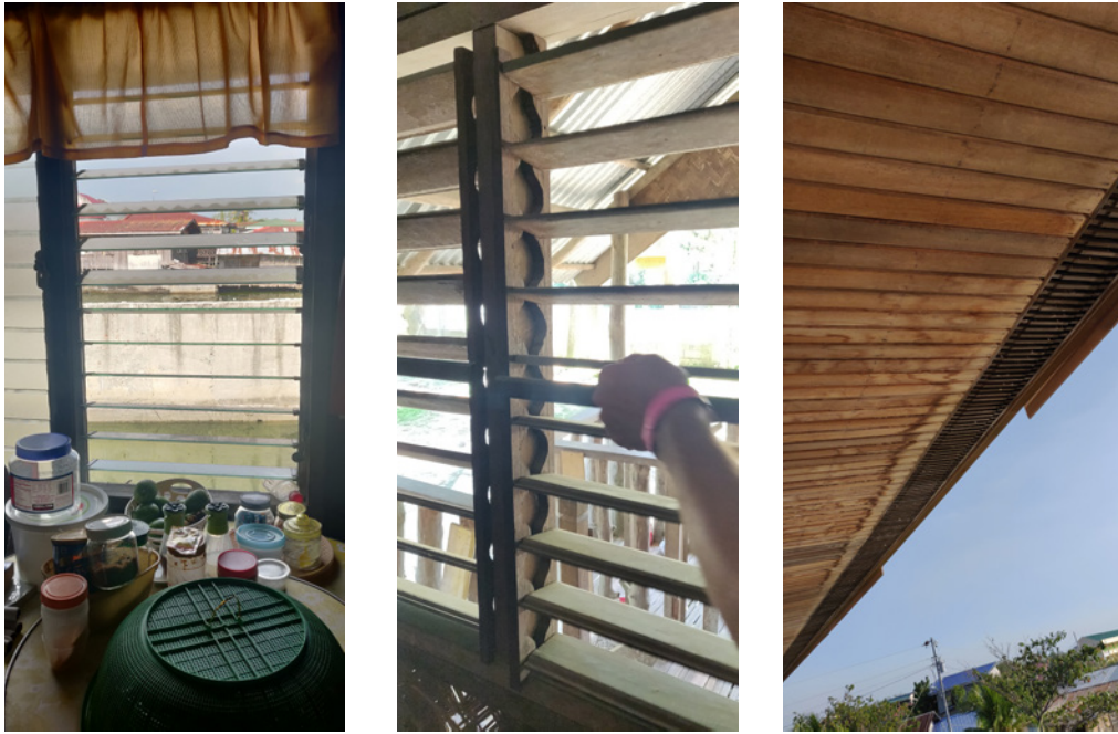
Figure 23: Operable glass louver in a residence, Hagonoy (left), operable wooden louver in a residence, Palawan (center) and roof ventilation in a residence, Macabebe (right)
