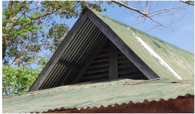
Figure 16: Louvered opening in roof, Palawan
