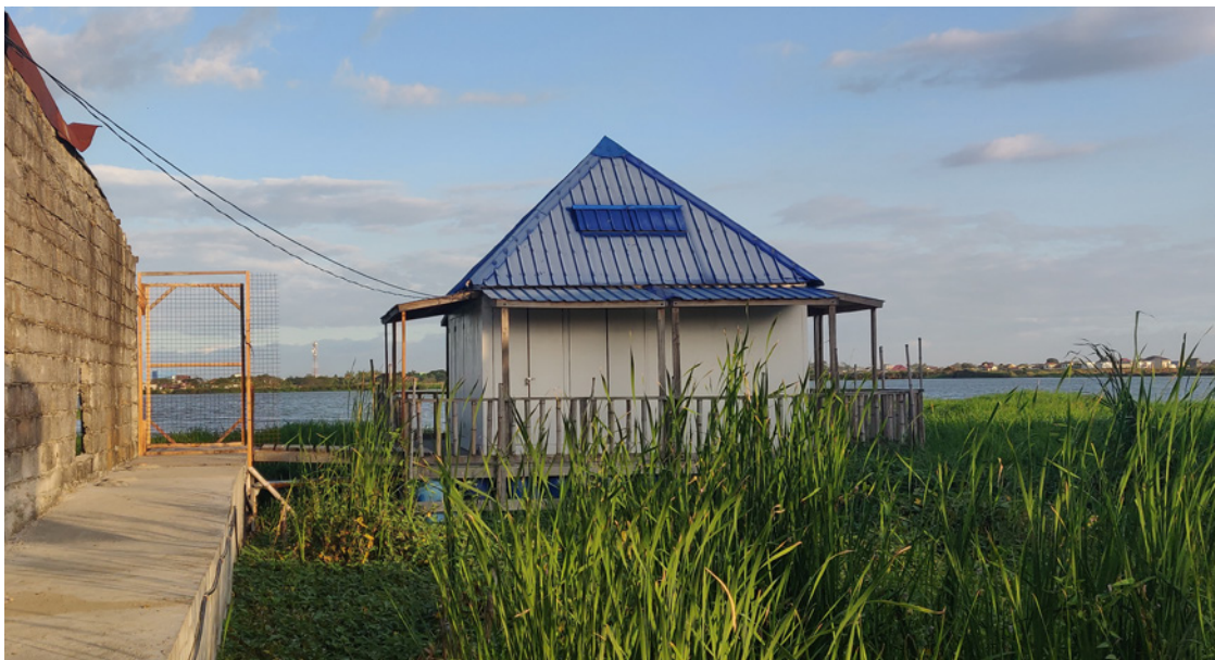
Figure 10: Floating house with newly made entrance gate and replaced poles supporting the eaves
