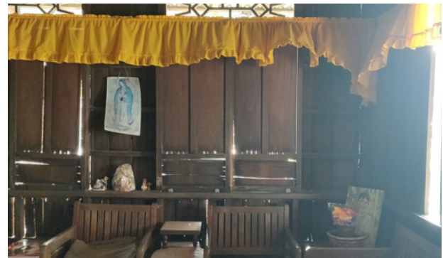
Figure 22: Ventilation below ceiling level, Hagonoy
