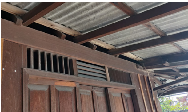
Figure 21: Ventilation below ceiling level, Hagonoy
