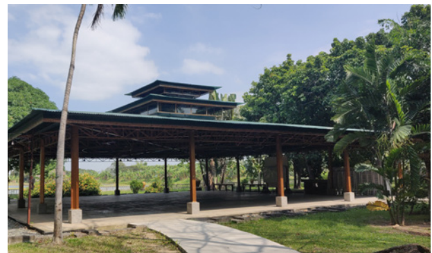
Figure 18: Open Hall with double roof, Hagonoy
