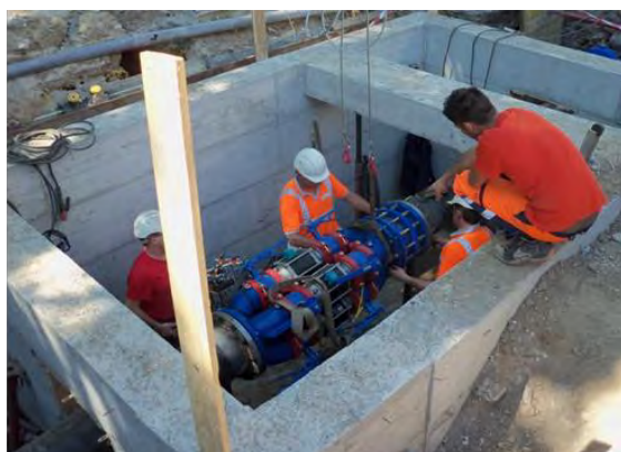
b. PRV chamber, from above
