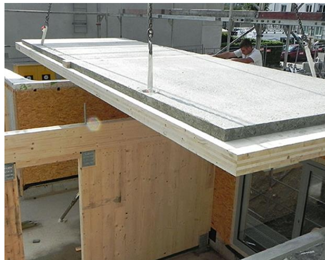
Figure 8: Prefab CLT-concrete composite floor (Vos & Jackson, 2024)
