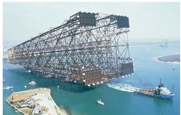
Figure 1.16: Largest jacket ever launched using a barge, the Bullwinkle jacket by Shell in 1989 which was over 500m long and weighed over 50,000 tons. Image is from: (ESA, 2011).
