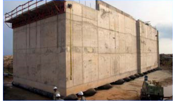
(b) Airbags used to transport a square concrete structure.
