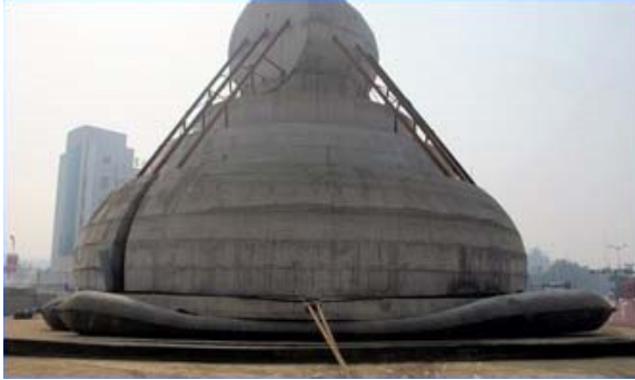
(a) Airbags transporting a round concrete structure
