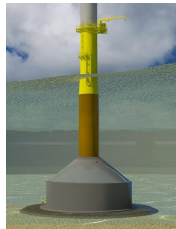
Figure 1.5: The concrete and steel conical GBF installed near Blyth. (Ten Oever & Overbeeke, 2017)
