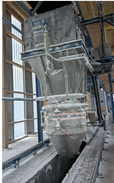
Figure 6.3: Dust suppression hopper at the warehouse
