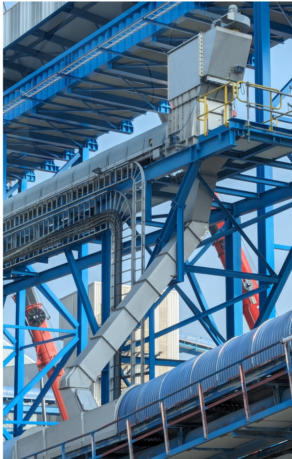
Figure 8.1: The considered transfer chute between two conveyor belts at Verbrugge
