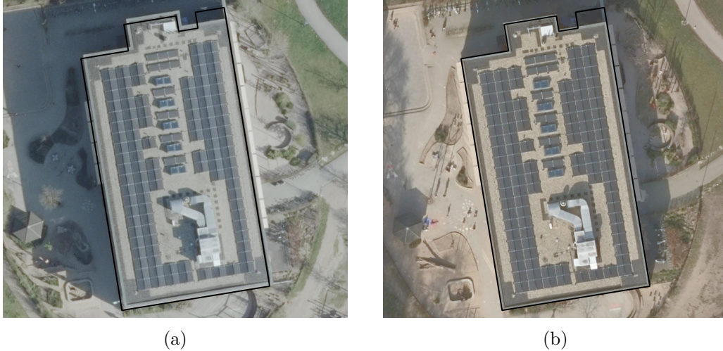
Figure 6: Example building footprint (i.e., the black polygon) superimposed on the corresponding 8 cm, true-color BM5 ortho- (a) and true orthoimagery 1 (b). There is significant data misalignment along the north side of the footprint.
