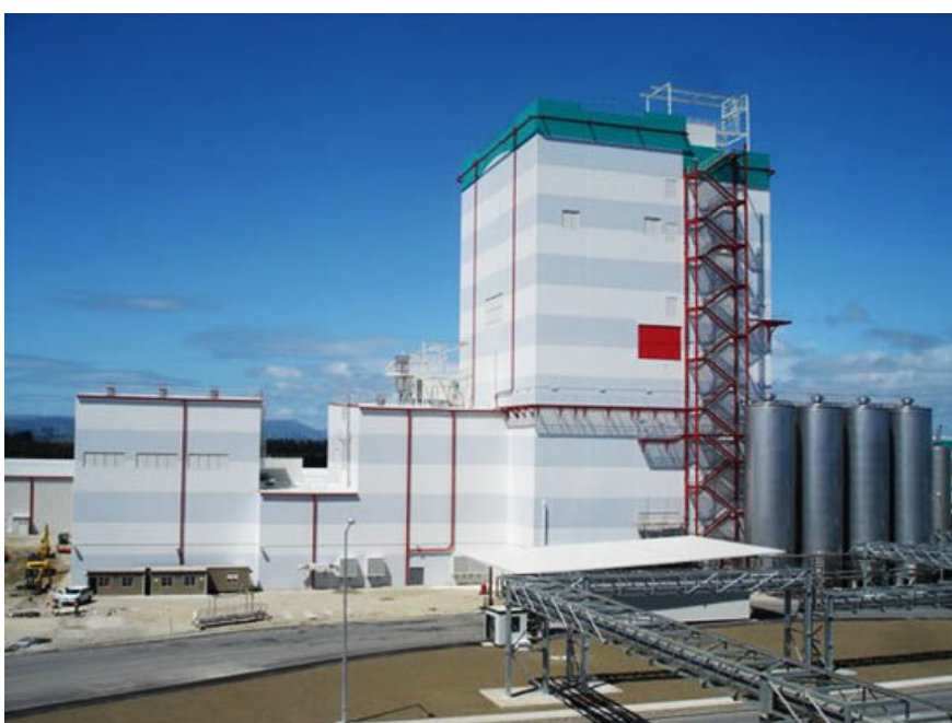
Figure 37 - Covered process installation
