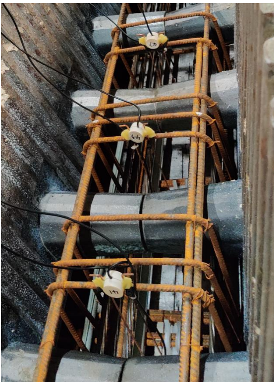
Figure 4-11: Picture of the precast girder formwork prior to casting
