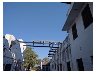
(b) Solar electricity panels for community
