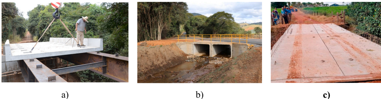
Fig. 6. Example of rural bridges commonly found in Brazil: (a) prefabricated two-way slabs for a composite bridge [34] (b) culvert bridge [35] and (c) prefabricated deck slab [36].
