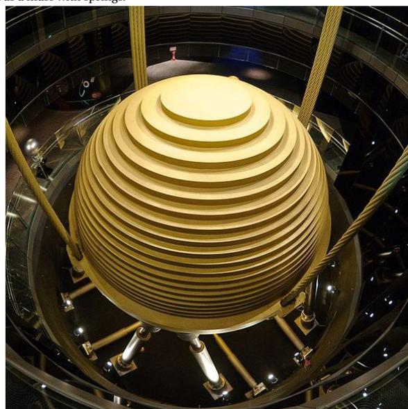
(d) The TMD in Taipei 101, Taiwan, which is implemented as a pendulum, but also is also attached from below by viscous dampers [1].
