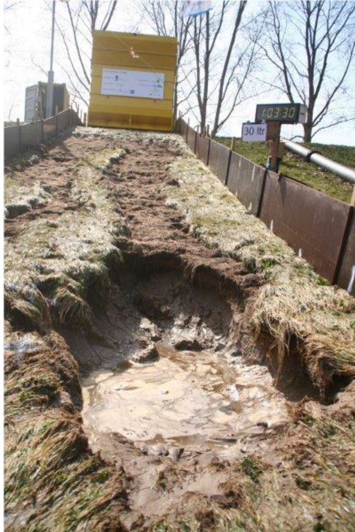
Figure A.13: Vechtdijk, test 3. Slope failure after incremental development. Damage started close to the crest, developed down slope as removal of grass layer and started to develop as a head-cut erosion at the lower half of the slope.
