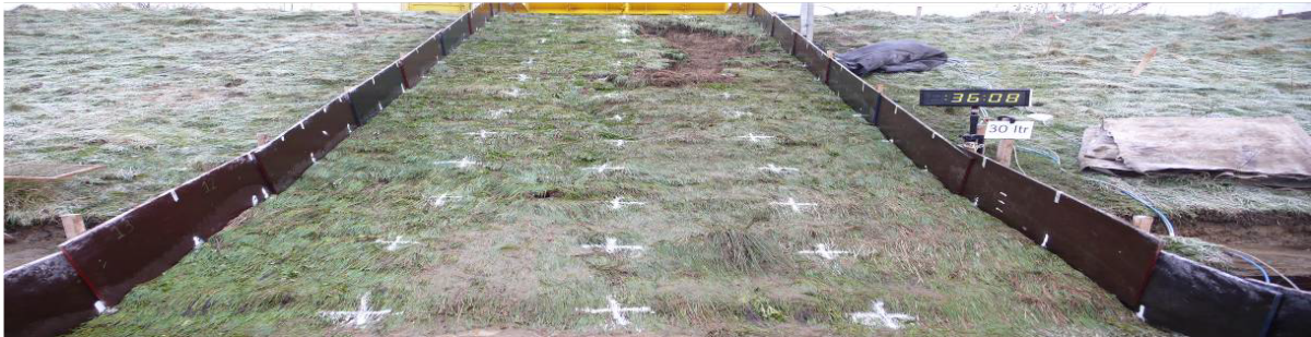
Figure A.10: Tielrode, section 1. Slope failure after 35 minutes simulation with a maximum load of 30 l/s/m overtopping waves. Start of failure of the slope cover close to the crest of the dike and developing downwards.
