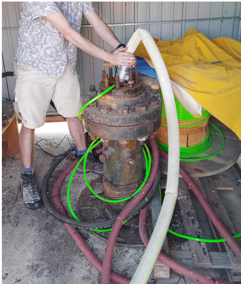
Figure 11: Well is being filled with river water from tank
