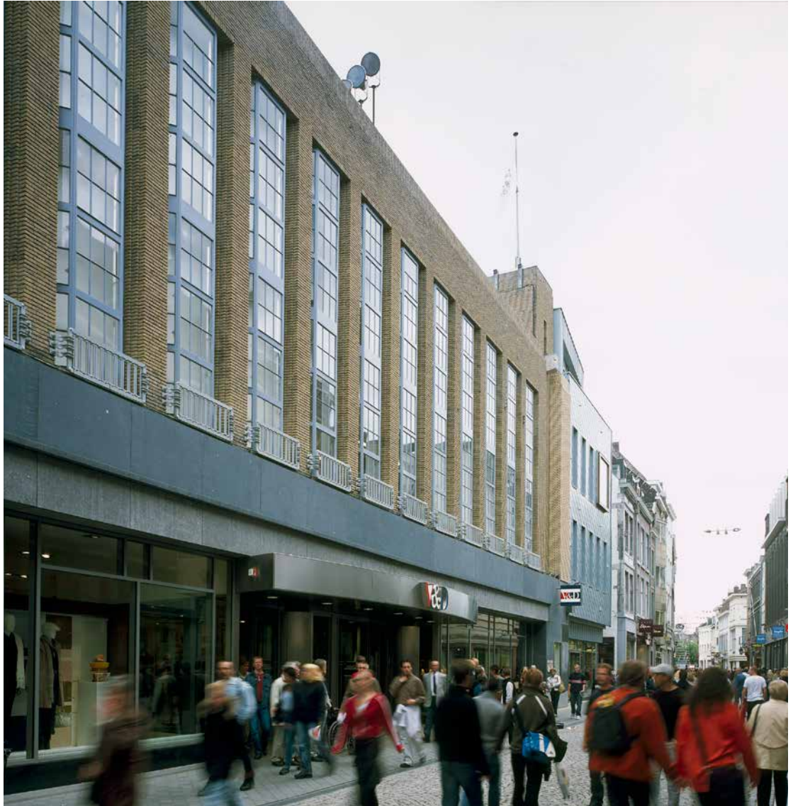
9. PHOTO OF THE CURRENT SITUATION OF THE GROTE STAAT FACADE
