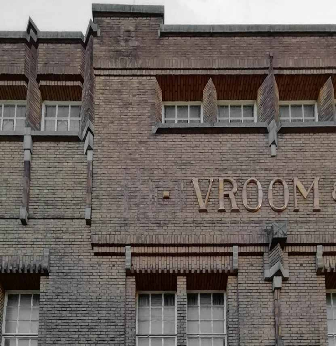
11. PHOTO OF THE CURRENT SITUATION OF THE LAAT FACADE
