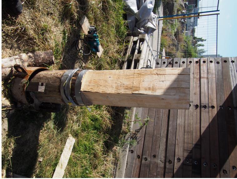
Figure G.5: Preparation Pile Head for Tensile Load Test
