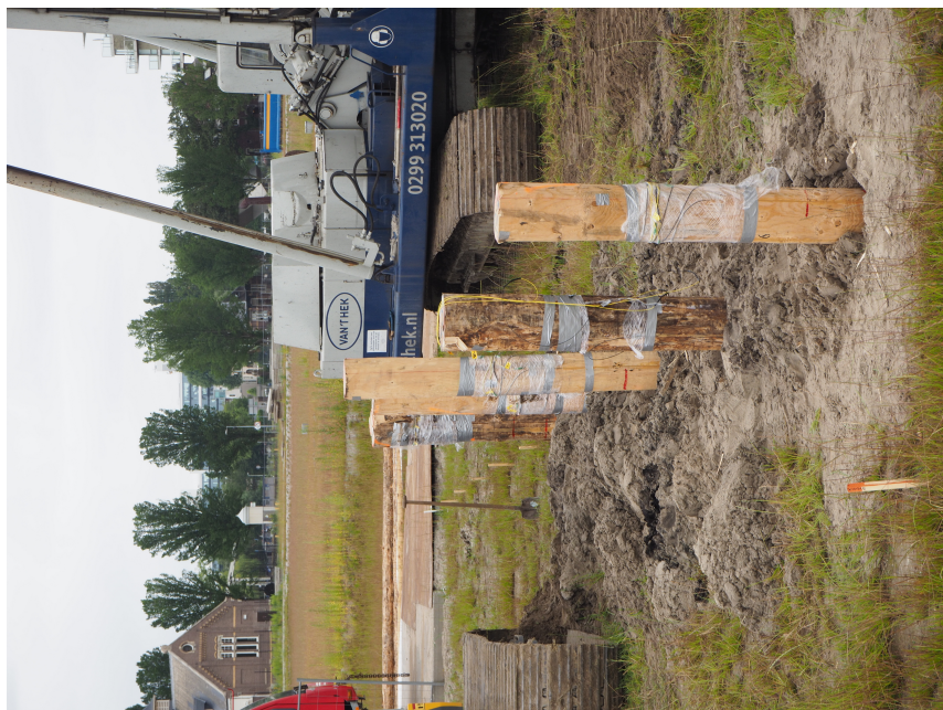
Figure G.4: Manually debarked (dark) and mechanically debarked (light) piles
