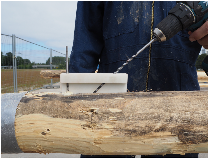
Figure G.1: Construction of Fiber Loop in Pile Tip
