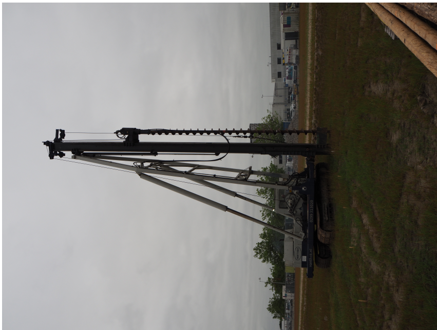
Figure G.2: Predrilling of Top Sand Layer
