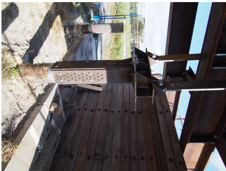
Figure G.6: Side view Tensile Load Test Set-Up
