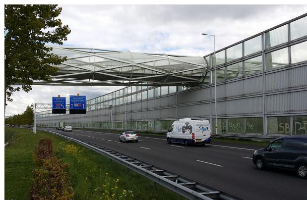
Fig. 10 A15 motorway with noise barrier and cyclist and pedestrian bridge
