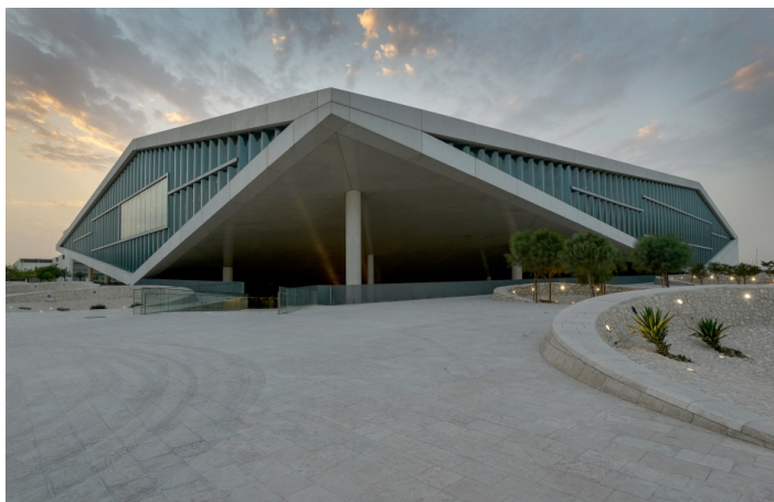
Figure 8. Façade National Library, Doha, Qatar
