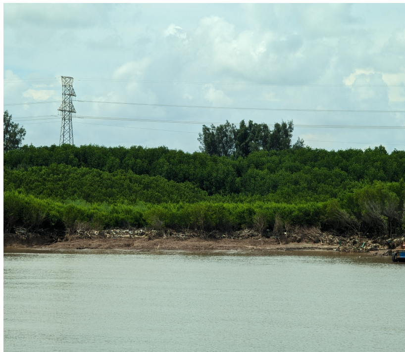
Figure A.2: The eroded part of the coast, east of Nha Mat, seen from the wind farm.
