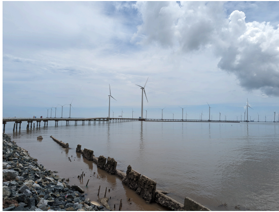
(a) The wind farm located at the eroded part of the coast of Bac Lieu.
