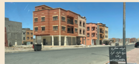
Figure 53: Photographs absence of vegetation cover in unfinished and finished areas.
