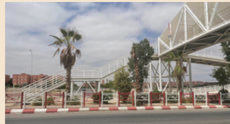
Figure 23: photograph pedestrian bridge main avenue Tamansourt
