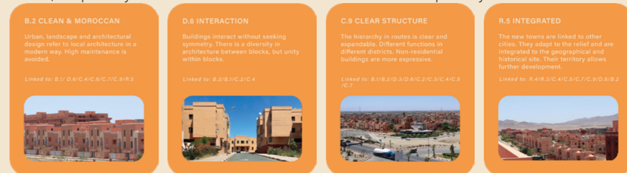
Figure 71: Al Omrane Pathway
