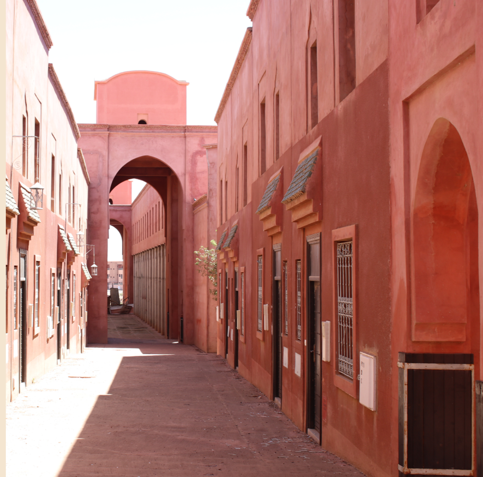
Figure 32: Photograph Tamansourt Medina. By author on 31 May 2022 >
