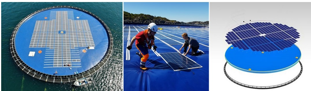
Figure 2.3: Pictures and sketch of the offshore solar power plant designed by Ocean Sun [46]
