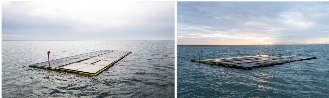
Figure 2.5: Impression of the offshore solar energy installation developed by Oceans of Energy and installed at the North Sea [47, 48]
