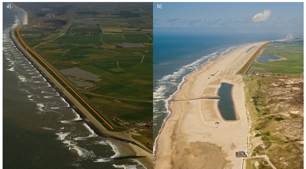
Figure 1. (a) Hondsbossche sea dike before placement of the nourishment (courtesy of Rijkswaterstaat, https://beeldbank.rws.nl/ , accessed on 6 September 2021) and (b) the Hondsbossche Dunes Nourishment just after placement in April 2015 (courtesy of Aannemerscombinatie Zwakke Schakel–Van Oord-Boskalis). The orange line marks the crest of the original sea dike.
