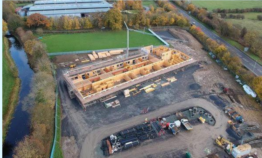
Aerial photo by Powys County Council
