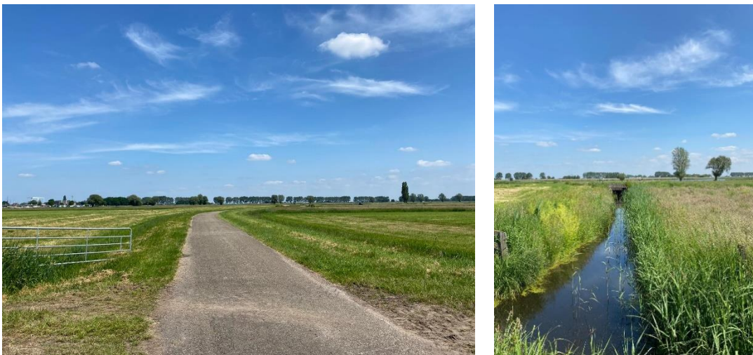
Figure A.7: Area located outside primary levees along het Zwarte Water near Genemuiden.
