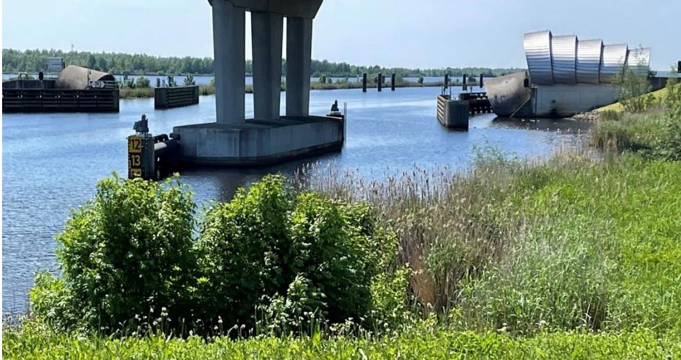
Figure A.6: Ramspol bellows weir.
