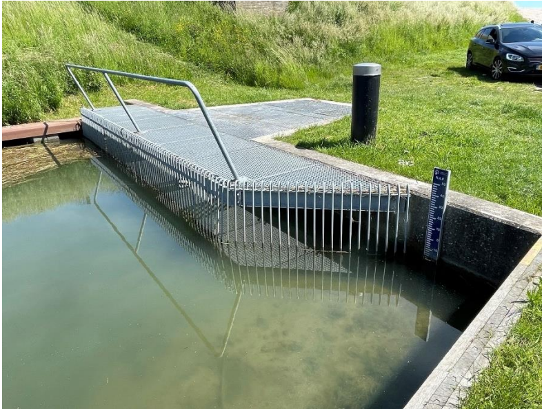
Figure A.4: Fence which catches duckweed in the nature area of Schellinkhout.
