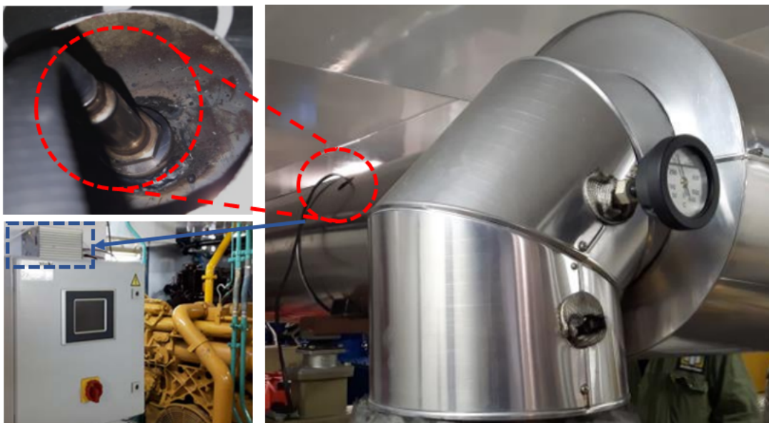
Figure 6.14: SEMS installed on an inland ship including \text{NO}_x sensor (own composition, 2018)
