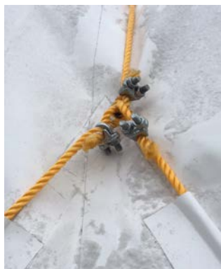
Figure 14: The joint connection of the cables
