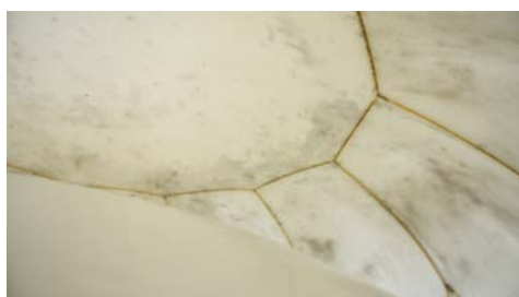
Figure 18: Removal of the inflatable mould
