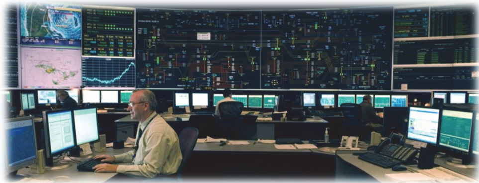
Figure 1.2: An example of a conventional SCADA-based control room, used by the power system operators to operate a power system (courtesy of IESO, Ontario).
