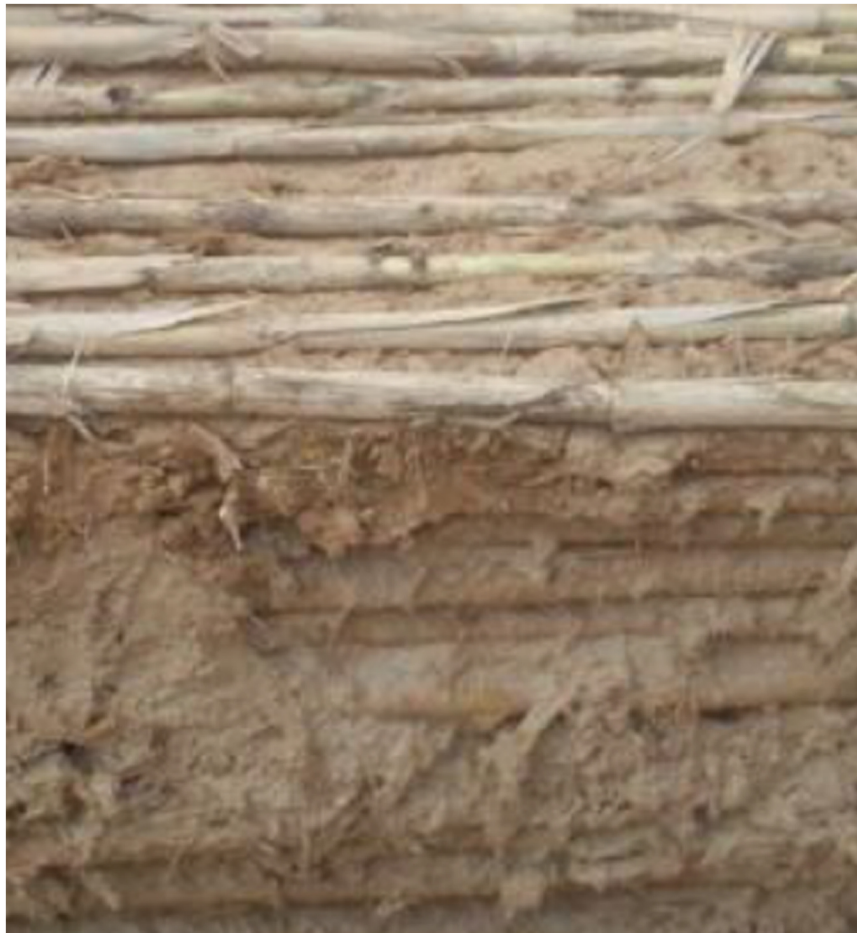
Figure 8. Easy to build monolithic wall made of layers of earth and reed fibre mortar and layers of reed, with simple framework (just to define vertical alignment) and wood pillars. From Energy efficiency. Performance of buildings (p. 19) , by Faria, P. & Ana, B., 2017, Research Gate.
