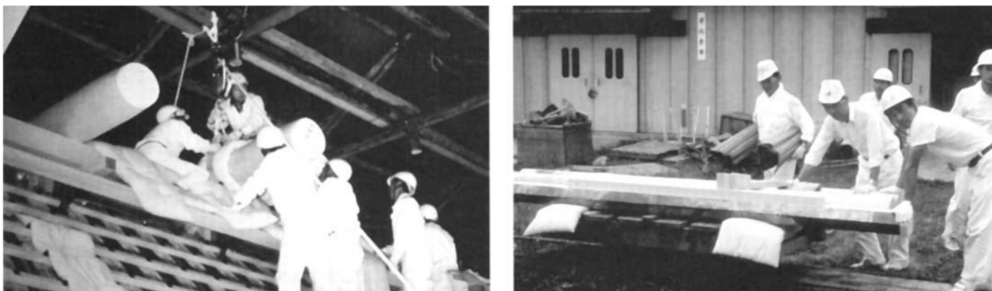
Image 1 (left): using a hand-operated winch for lifting heavy wooden members into place (Adams, 1998). Image 2 (right): trolley for moving materials from the work yard to the sacred building site (Adams, 1998).
