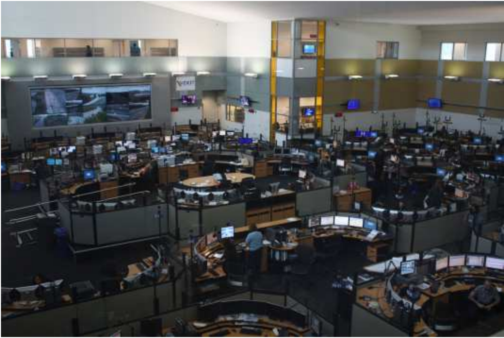
Figure 8: VDOT Traffic Control Center
