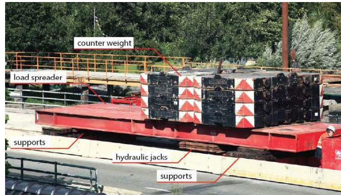
Fig. 3. Photograph of proof loading configuration as used by DUT
