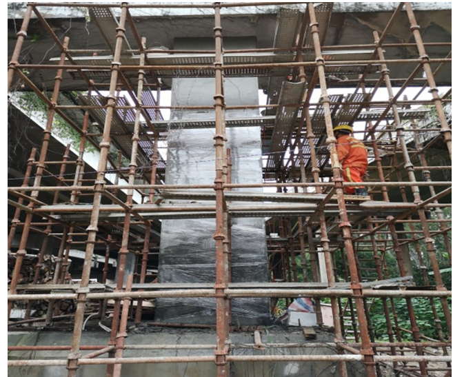
FIGURE 2 Installation of impressed current cathodic protection-structural strengthening (ICCP-SS) system on piers of the Guangzhou-Shenzhen highway
