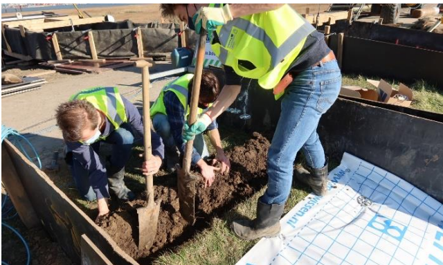
Figure 20 Digging trench upper damage (keeping grass layer intact by flipping it)
