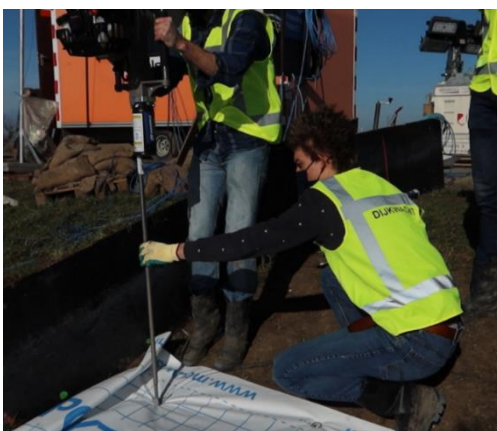
Figure 16 Drilling TL-DTOOL anchor installation rod at start of drilling phase
