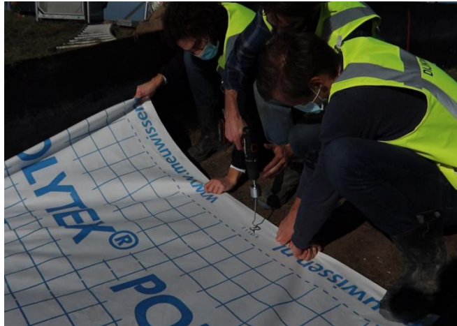
Figure 14 Installation of pins with the drill with Gripple attachment
