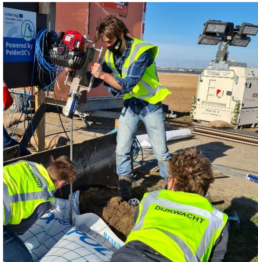
Figure 3 Drilling of TL-DTOOL anchor installation rod with GPD (plastic sheet in figure is Polytex®, not Tyvek®)
