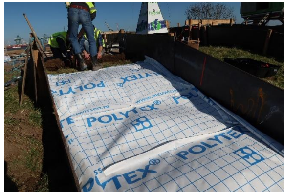
Figure 19 Placed sheets at upper damage
