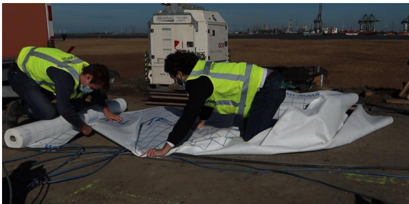
Figure 13 Cutting of plastic sheets at top of dike in windy conditions
