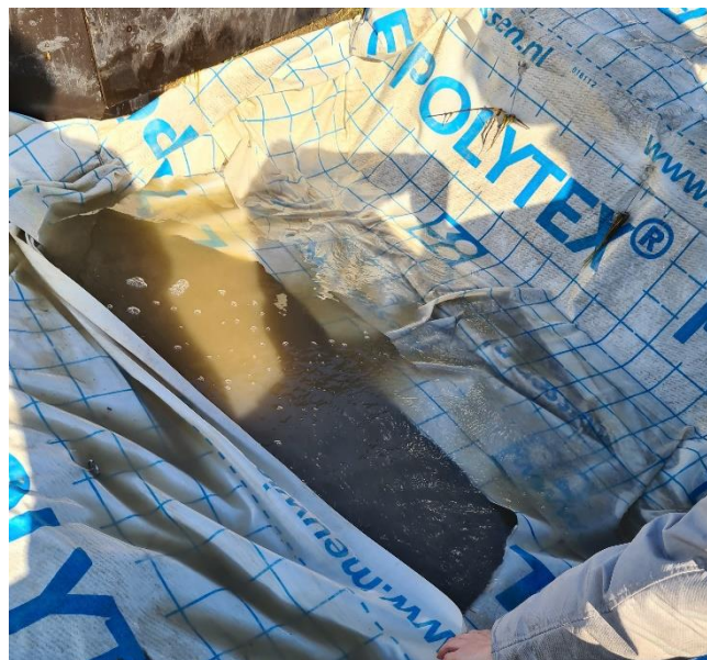
Figure 34 Torn off sheet at lower damage after tear was made
