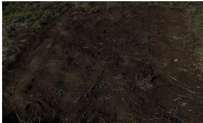
Figure 27 Upper damage after removing repair solution after all overflow were performed
