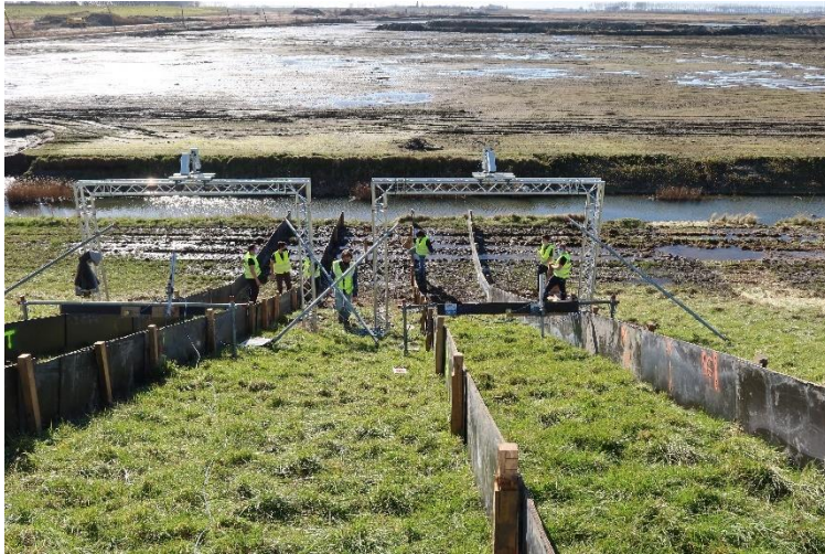
Figure 8 Measuring equipment on test strip dike
