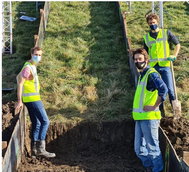
Figure 11 Lower damage test strip
