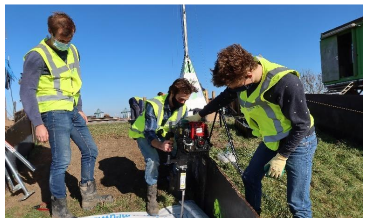
Figure 15 Drilling TL-DTOOL anchor installation rod at almost end of drilling phase
