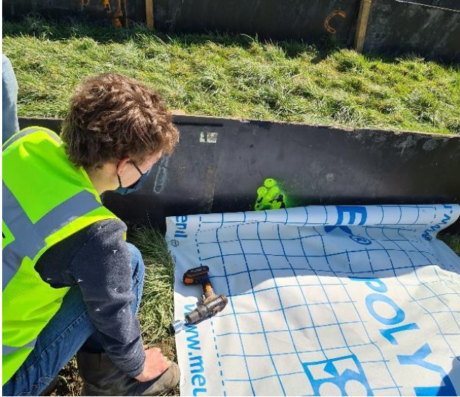
Figure 32 Double folded sheet at side of the test strip
