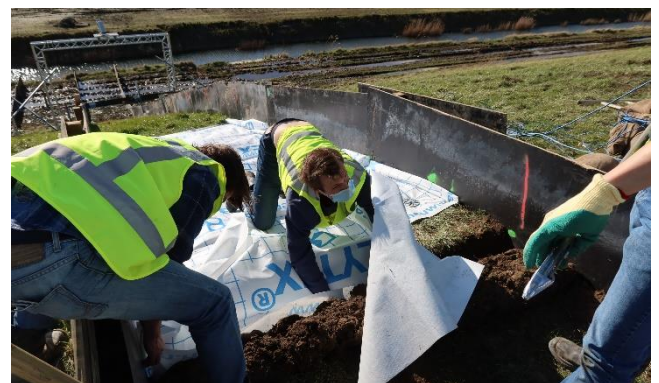
Figure 21 Putting upper sheet into trench at upper damage
