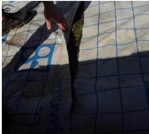
Figure 26 1m tear through two layers sheet at lower damage
