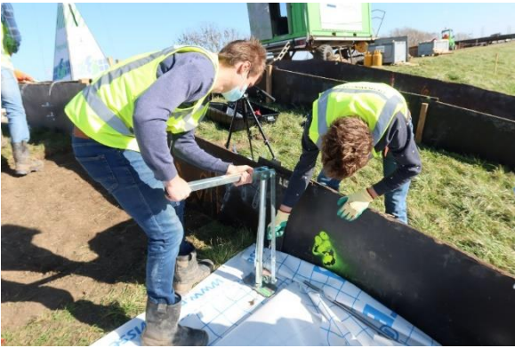
Figure 18 Tightening the anchor with JackJaw®
