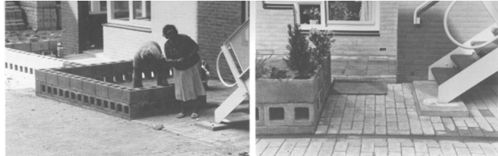
the small concrete bloc wall;
