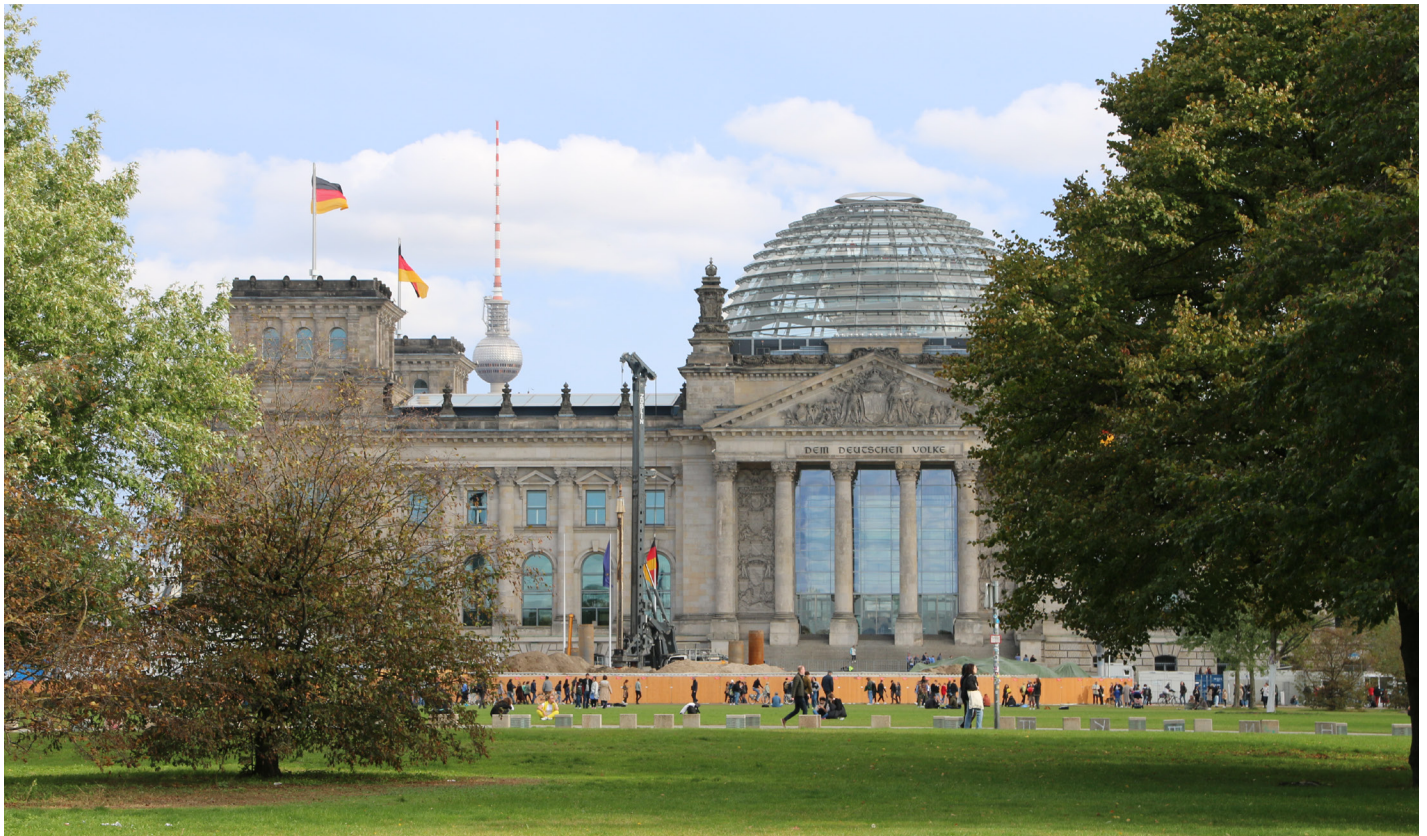
Figure 011: The old Reichstag Building photographed from the exact location where the new Adaptable Bundestag Complex will be built.
