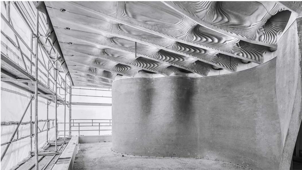
*Figure 1-22: The DFAB House Smart Slab During Construction, Source: NCCR Digital Fabrication*
