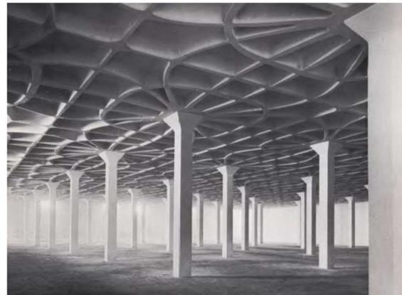
Figure 1-1: Gatti Wool Factory Floor System (Halpern, et al., 2013)
