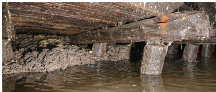
Figure 2.4: Foundation of Amsterdam quay walls(Gemeente Amsterdam, 2019a)
