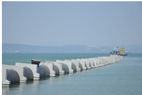
Figure 4.3: Ballasted HDPE Pipeline [49]
