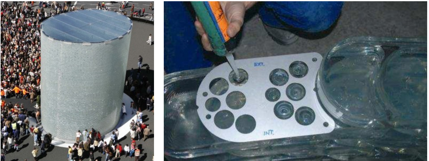
Figure 5.3: Atocha memorial building (left) and distribution of glue on the brick (right). Retrieved from Bellapart & Sau (n.d.).
