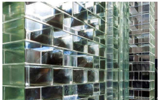
Figure 4.9: Cast glass façade for the Chanel Crystal house in Amsterdam. Retrieved from ABT (2016).
