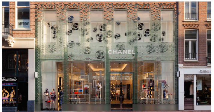
Figure 1.4: Cast glass façade for the Chanel Crystal house in Amsterdam. Retrieved from ABT (2016).
