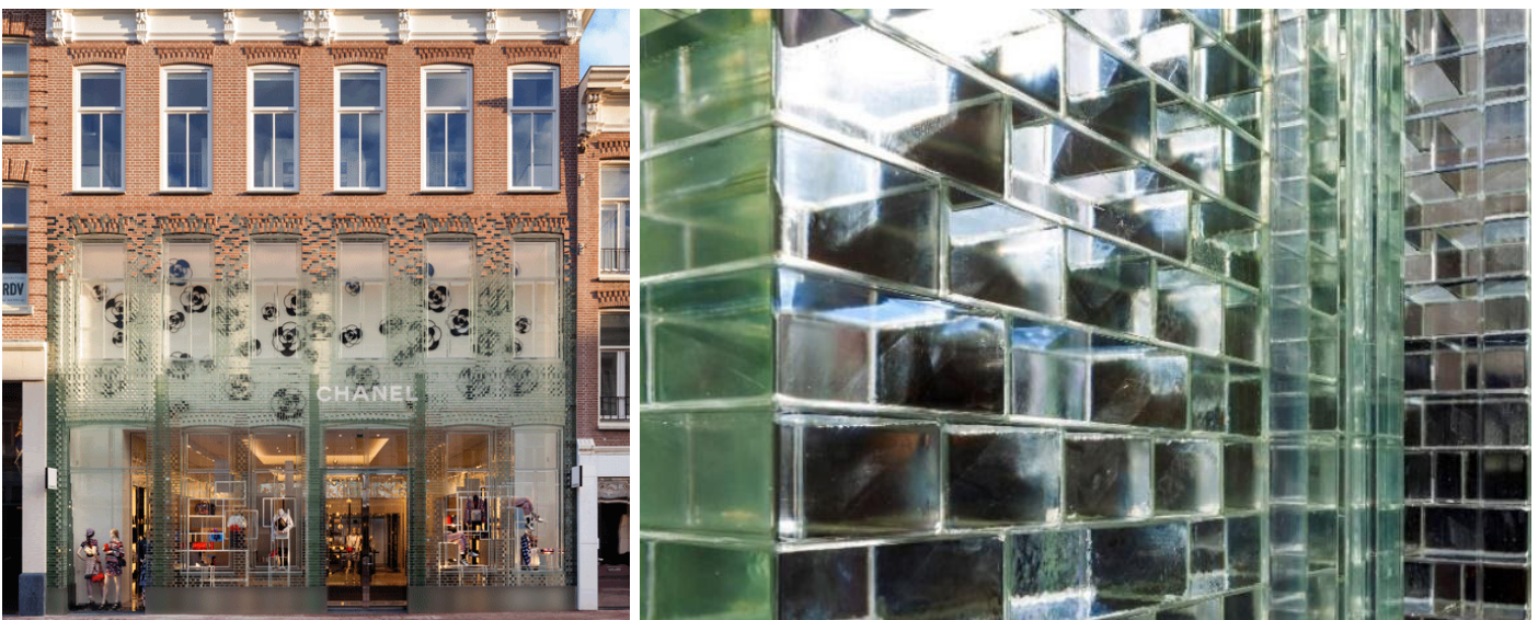
Figure 5.4: Cast glass façade for the Chanel Crystal house in Amsterdam. Retrieved from ABT (2016).
