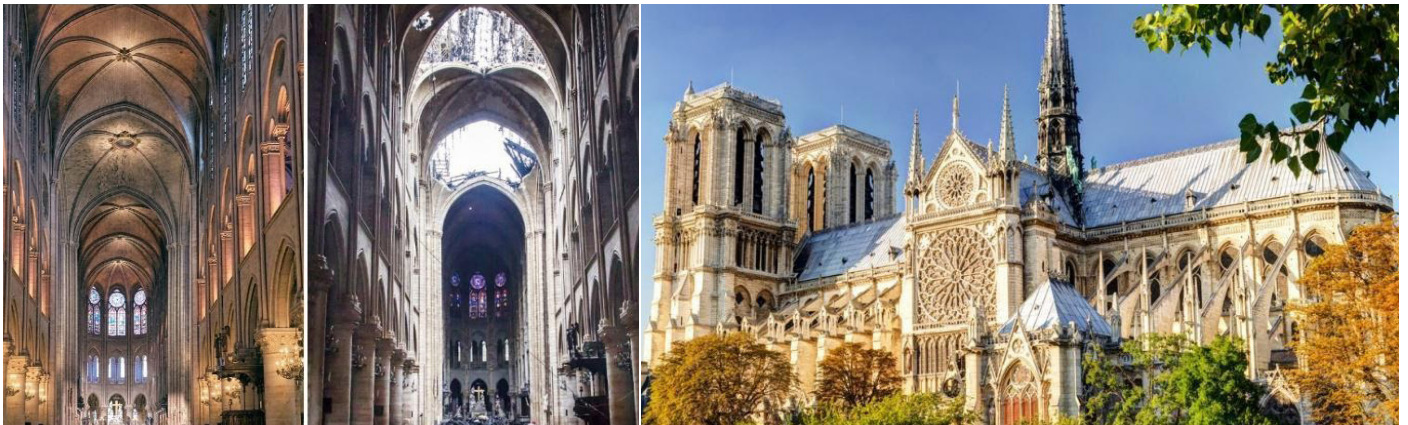
Figure 1.5: Interior before the fire (left), Interior after the fire (middle) and exterior before the fire (right). Retrieved from Shaw (2019).
