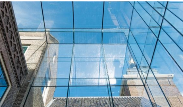
Figure 1.3: Glass roof structure (Castle Ruurlo). Retrieved from Verlaan&Bouwstra (2013).
