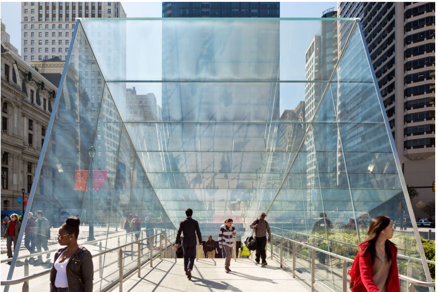
Figure 4.4: Structural float glass panels as metro entrance. Retrieved from EOC Engineers (n.d.).
