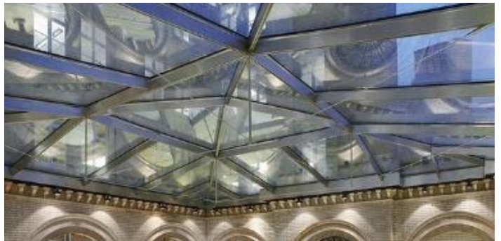
Figure 1.2: Steel roof structure (Apple store). Retrieved from Worldarchitecturenews (2011).
