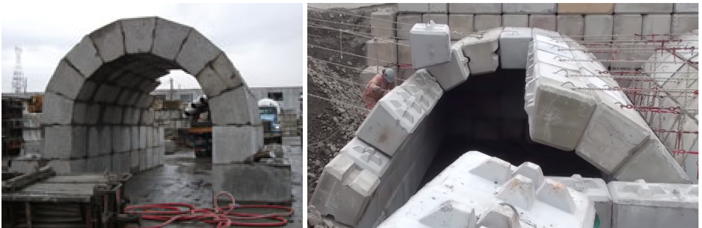
Figure 5.10: Interlocking system for a concrete vault. Retrieved from Lockblock (n.d.).
