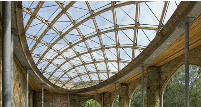
Figure 1.1: Wooden roof structure (Chiddingstone Orangery Castle). Retrieved from Carpenteroak (2007).
