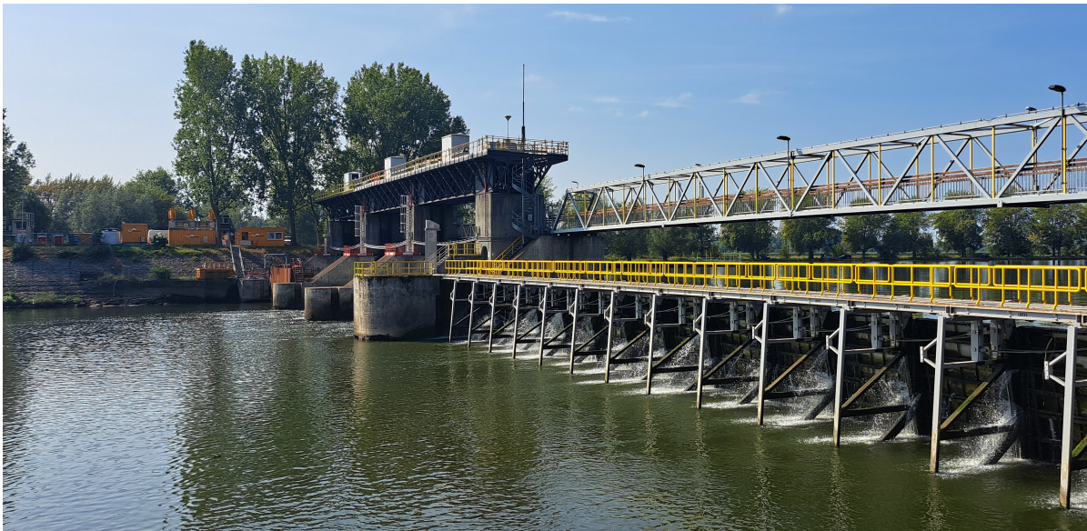
Figure 3.1: Photo of the Linne weir with the Poirée section in the front (right side) and the Stoney section in the back (left side).
