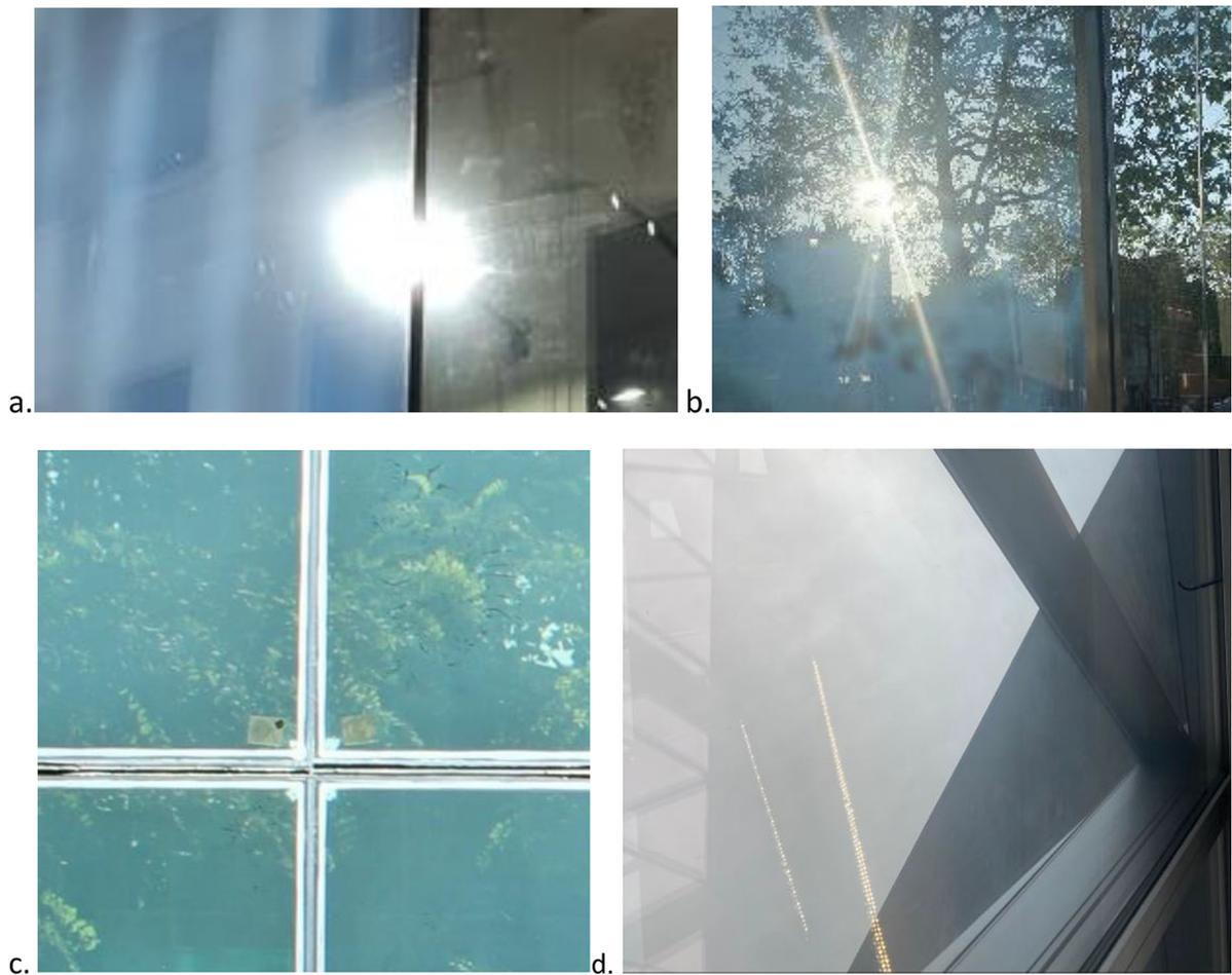
**Fig. 1** Examples of visual defects related to view clarity in a few recent new façade and glazing assemblies: **a** haze defect due to interlayer performance at night under artificial lights; **b** haze defect under daylight conditions. **c** view clarity defect due to novel responsive electrochromic layers; **d** view clarity defect due to fogginess in close cavity assemblies
