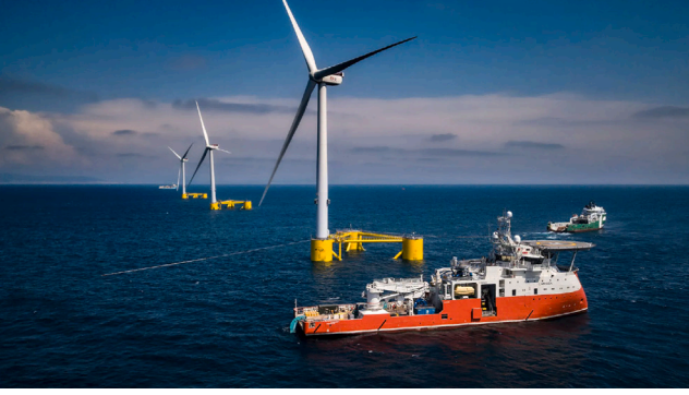
Fig. 1. Support vessel and wind turbine, resp. a planar and tubular maritime structure.
